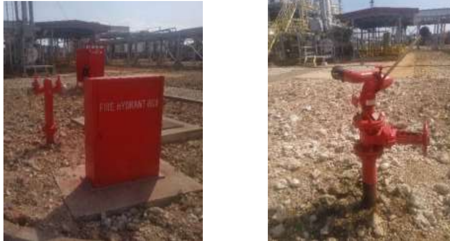
Figure 9: Fire hydrant and fire monitors
