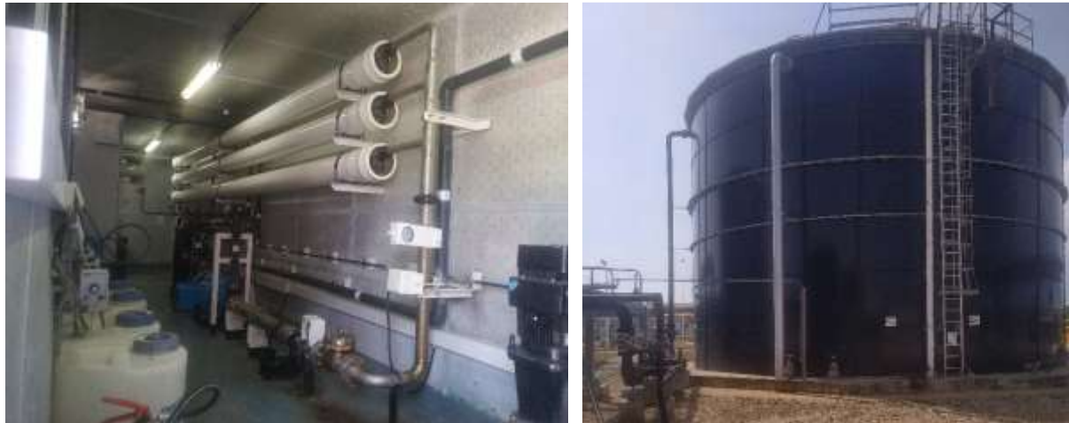
Figure 4: Reverse Osmosis unit for portable Water Treatment & Storage tank
